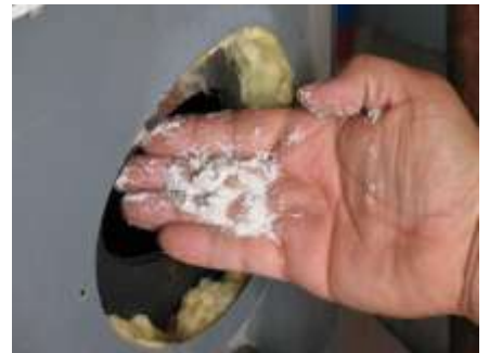
Installed 2/21/07 – room #27 still in service
